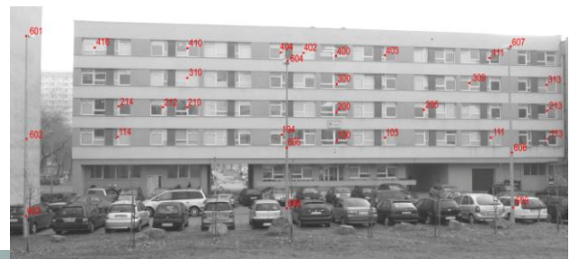
Figure 2. Test field #1 – building façade
