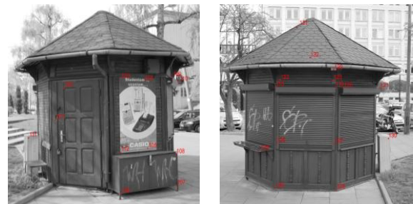
Figure 3. Test fields #2 – small building
